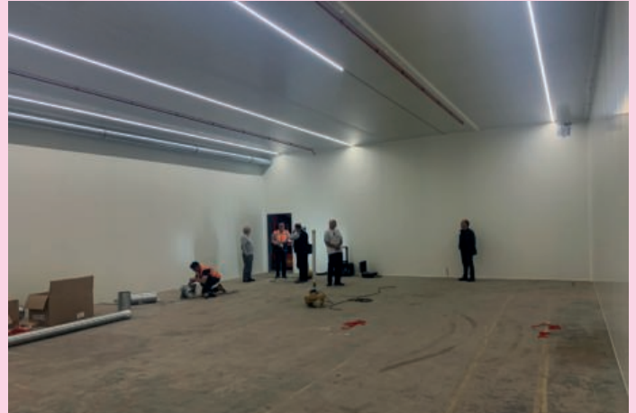
The storage pod is constructed to give minimal heat changes and precise control of humidity. It also gives good fire protection.
