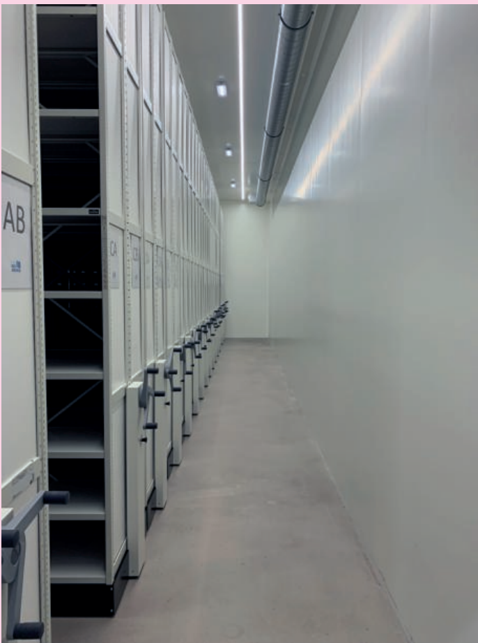
The pod now with high density rolling racking installed.
