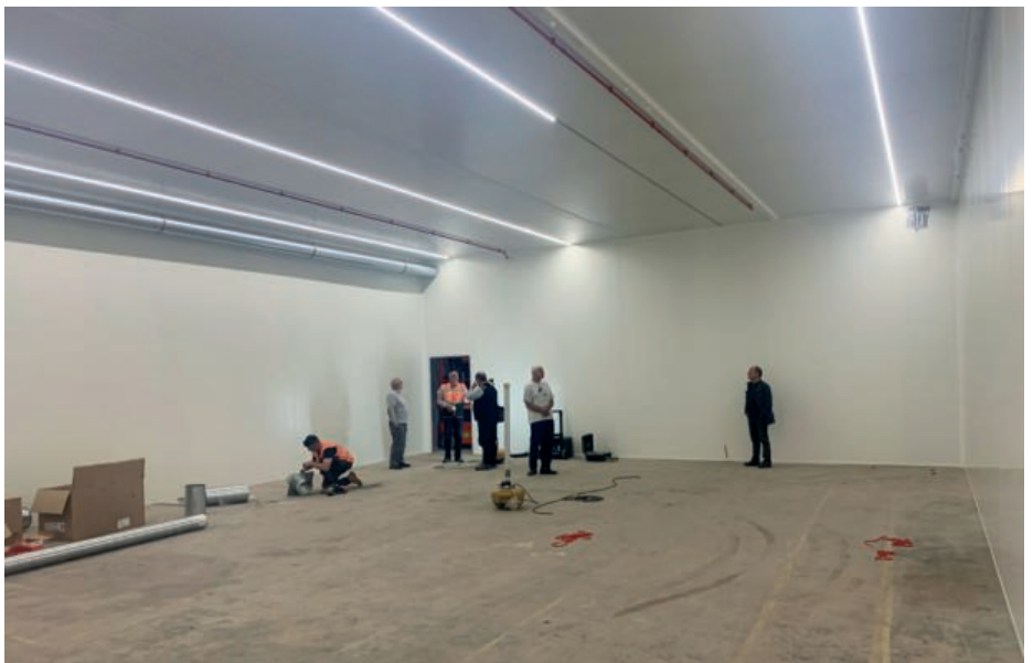
The storage pod takes shape.
