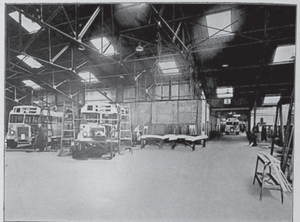
Final stages of body completion and panel mounting.
