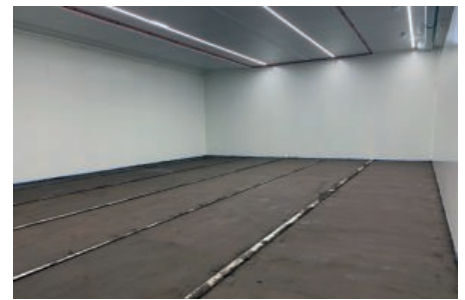
Screed and shelving rails in place.
