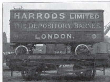
FIG. 5.—Tying the Wheels of a Furniture Van.
